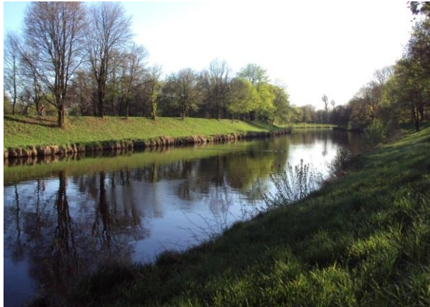
Fig. 3: Regulated part of the stream in the built-up area of Hradec Králové (photo M. Vávra, 28. 4. 2014)
