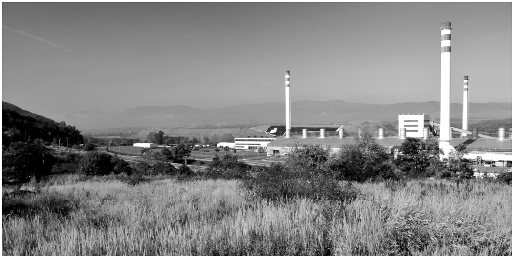
Fig. 6: Aluminium plant and the waste dump in Žiar nad Hronom in the Žiarska Kotlina basin (study area 5)
