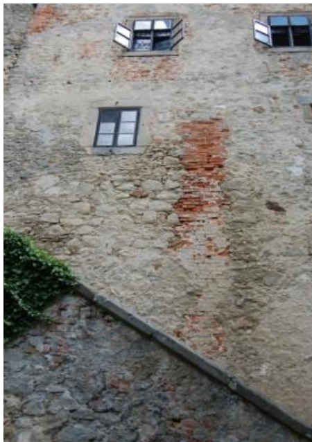
Fig. 2: A walled-in shaft leading from a toilet to the second courtyard at Buchlov Castle, autor: F. Havlíček (2016)
