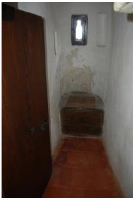
Fig. 6: The interior of a fortified toilet (Buchlov Castle), author: F. Havlíček (2016)
