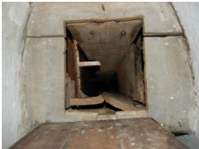
Fig. 8: Detail of the toilet drainage system (Buchlov Castle), author: F. Havlíček (2016)
